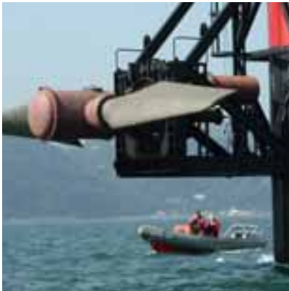
'Seaflow' tidal power generator off Lynmouth, with generator, rotor and collar raised above water.
