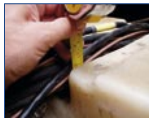
Photograph 2: The configuration in another Warrior configured as expected, providing the required deeper space for installation of cabling.
