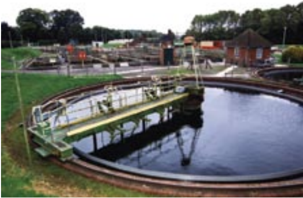
Views of the Tidworth Sewerage works.
