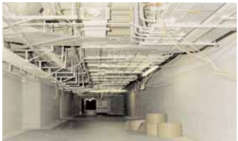
Photographs showing the complexities of the mechanical and electrical engineering works
