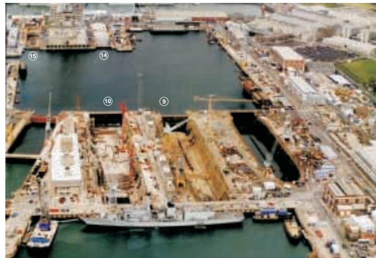
Aerial view of No 5 basin looking north showing the largest dry docks at Devonport Royal Dockyard. The D154 project embraces the upgrade of the middle dry dock (No 9), together with the two dry docks (Nos 14 and 15) partially visible in the top left hand corner of the photograph. Upgrade work is also underway on No 10 dock, on the left of the photograph.
