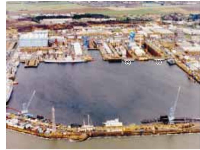
Aerial view of the main basin at Rosyth Royal Dockyard looking north. The existing submarine refit complex is between the two dry docks (Nos 2 and 3) in the top right. The ship lift and refit sheds are in the top left.
