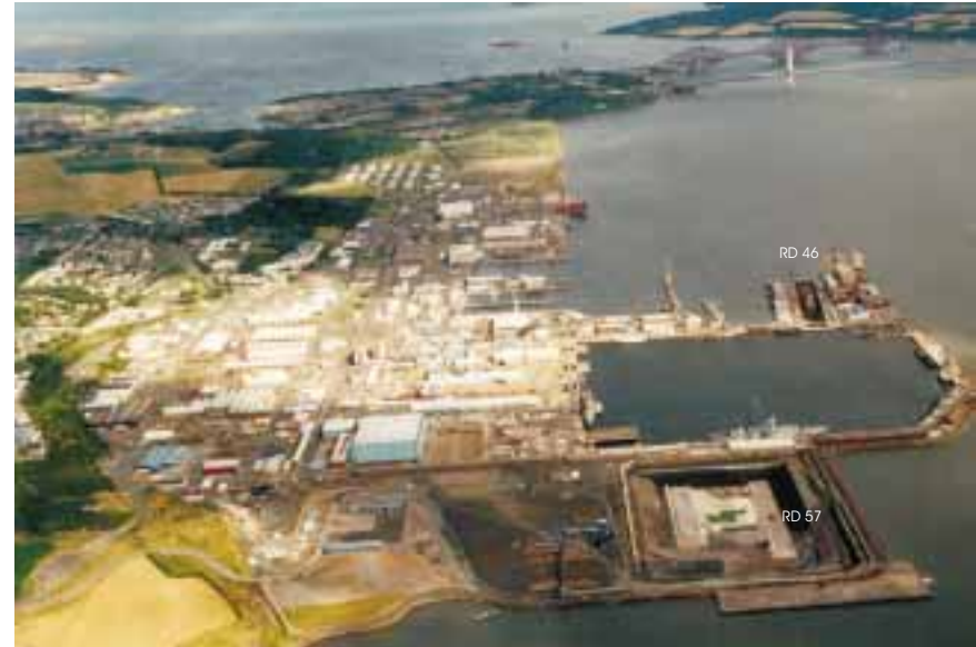
Aerial view of Rosyth Royal Dockyard looking east towards the Forth Road and Rail bridges. The photograph shows the main basin, the entrance lock (RD 46), and the large excavations which were part of the discontinued RD 57 project.
