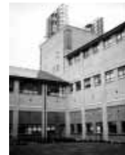
Courtyard and ventilation from fume cupboards
