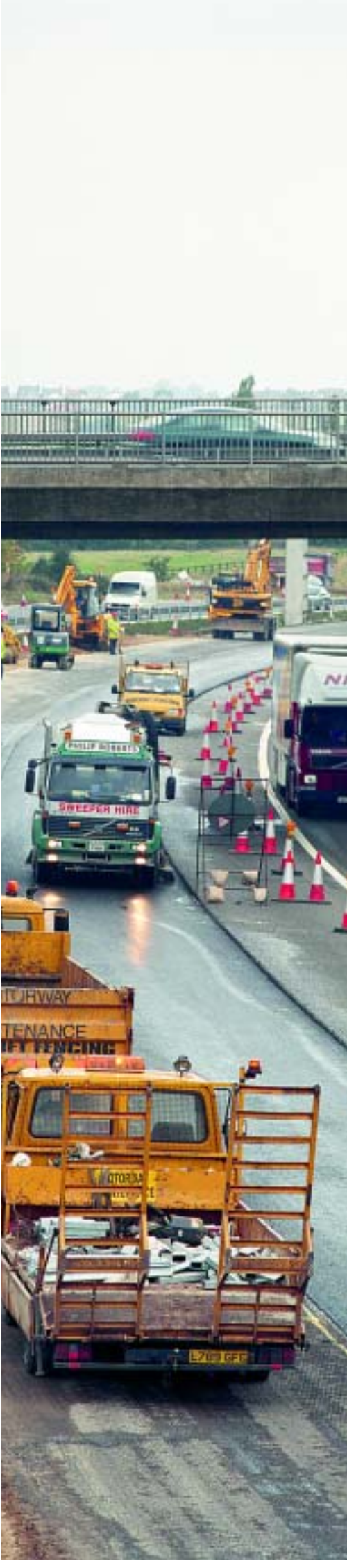
M1 Junction 28 contraflows and roadworks, October 2000
