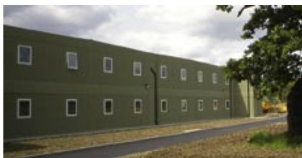
**Modular temporary units** are prefabricated two-story buildings, similar to portacabins. Each unit provides 40 cells, separate communal toilet and washing facilities, an association room, a food servery, and staff office.
