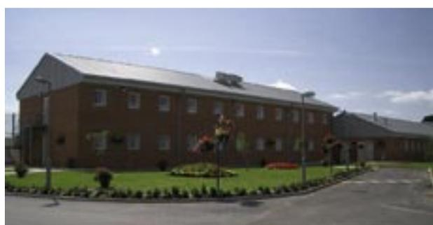
**Brick-clad steel framed units**, are based on the on-shore accommodation units used in oil fields. The units are primarily manufactured off-site with erection and completion taking place on site. A standard unit has 40 cells each with its own sanitary facilities.
