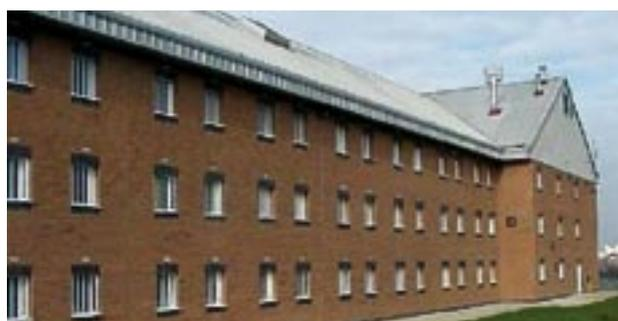
**Houseblocks** are standard prison accommodation constructed from either reinforced concrete or built from steel modular units. New houseblocks can be built in existing prisons.
