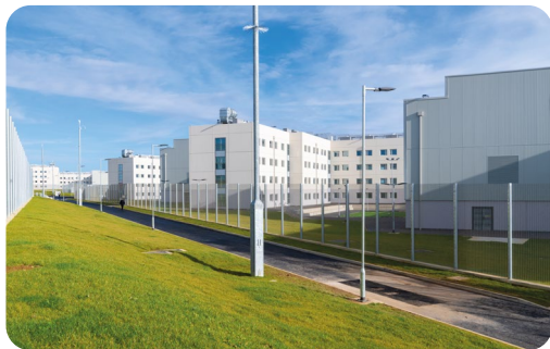
New build prison wings, HMP Five Wells
