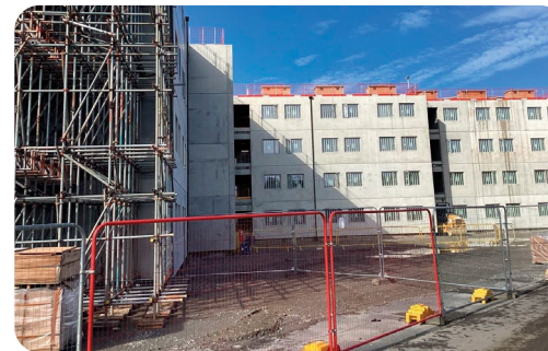
Accelerated houseblock construction, HMP Elmley
